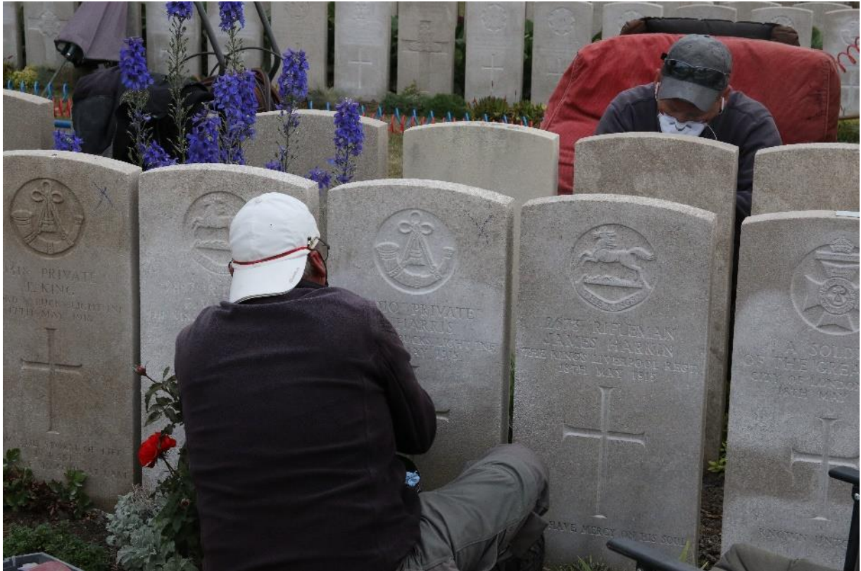
Headstone re-engraving being done in one of the cemeteries maintained by the CWGC ©CWGC
